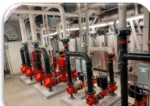
Assumption HVAC Upgrade
